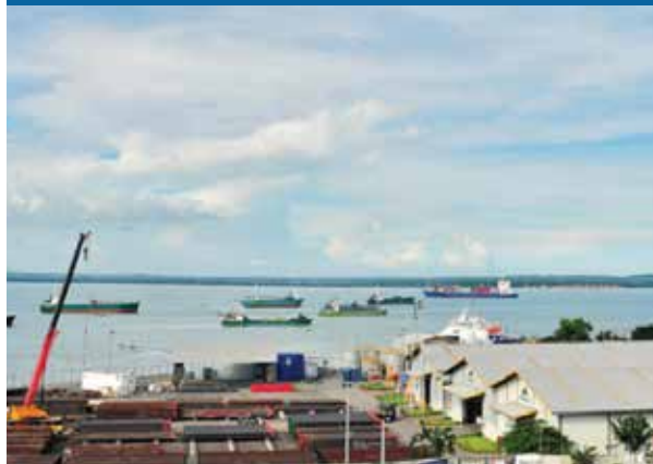
PIPE RACKING, FUEL TANKS AND WAREHOUSES
