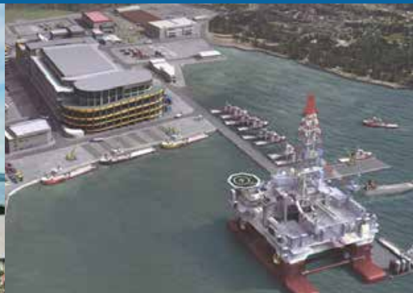
OIL RIGS PARKING FOR SUPPLY/MAINTENANCE
