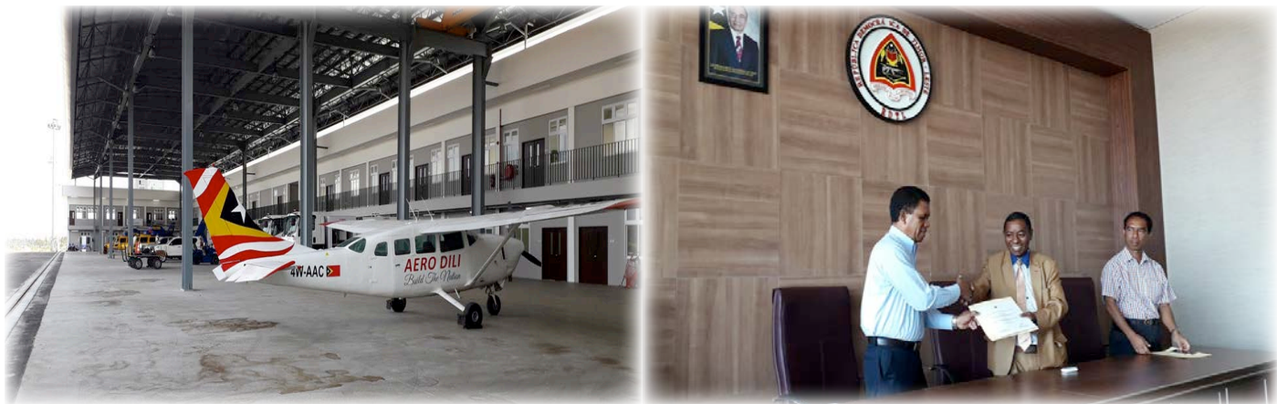
Figure 4-7: Hangar helicopter with capacity for 4 units helicopter and 1 unit overhead crane at maintenance area, with a length of 106.8m and 22m wide (left); Suai Airport partial hand over to ANATL (right)
