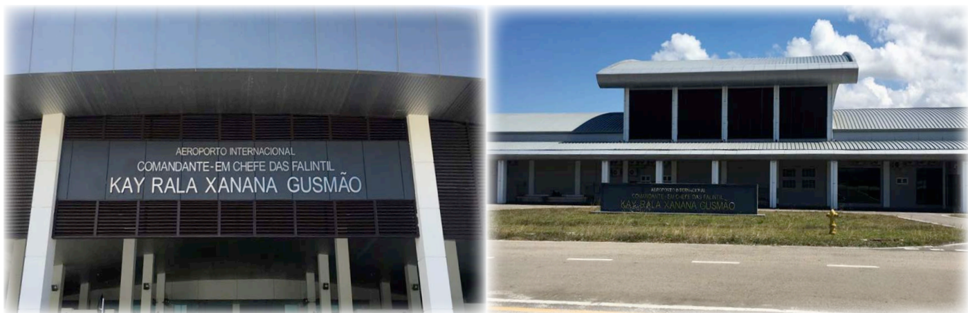
Figure 4-5: Main façade of the new terminal building
