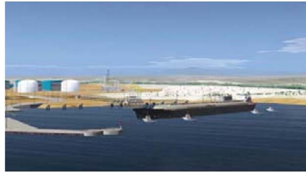
Marine facility for the TLNG project
