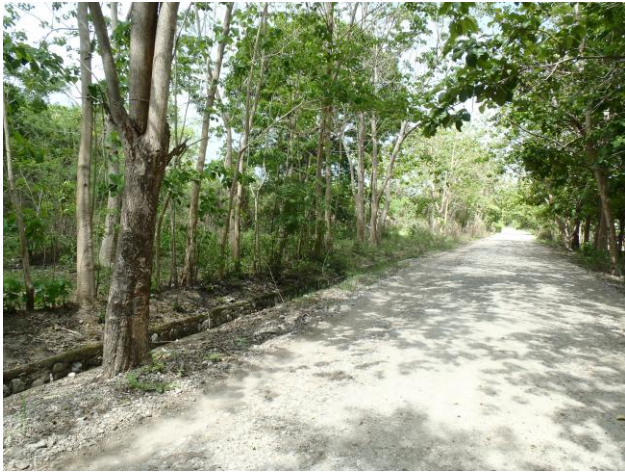
Plate 7-18 on Figure 7-17 (looking north-west)
