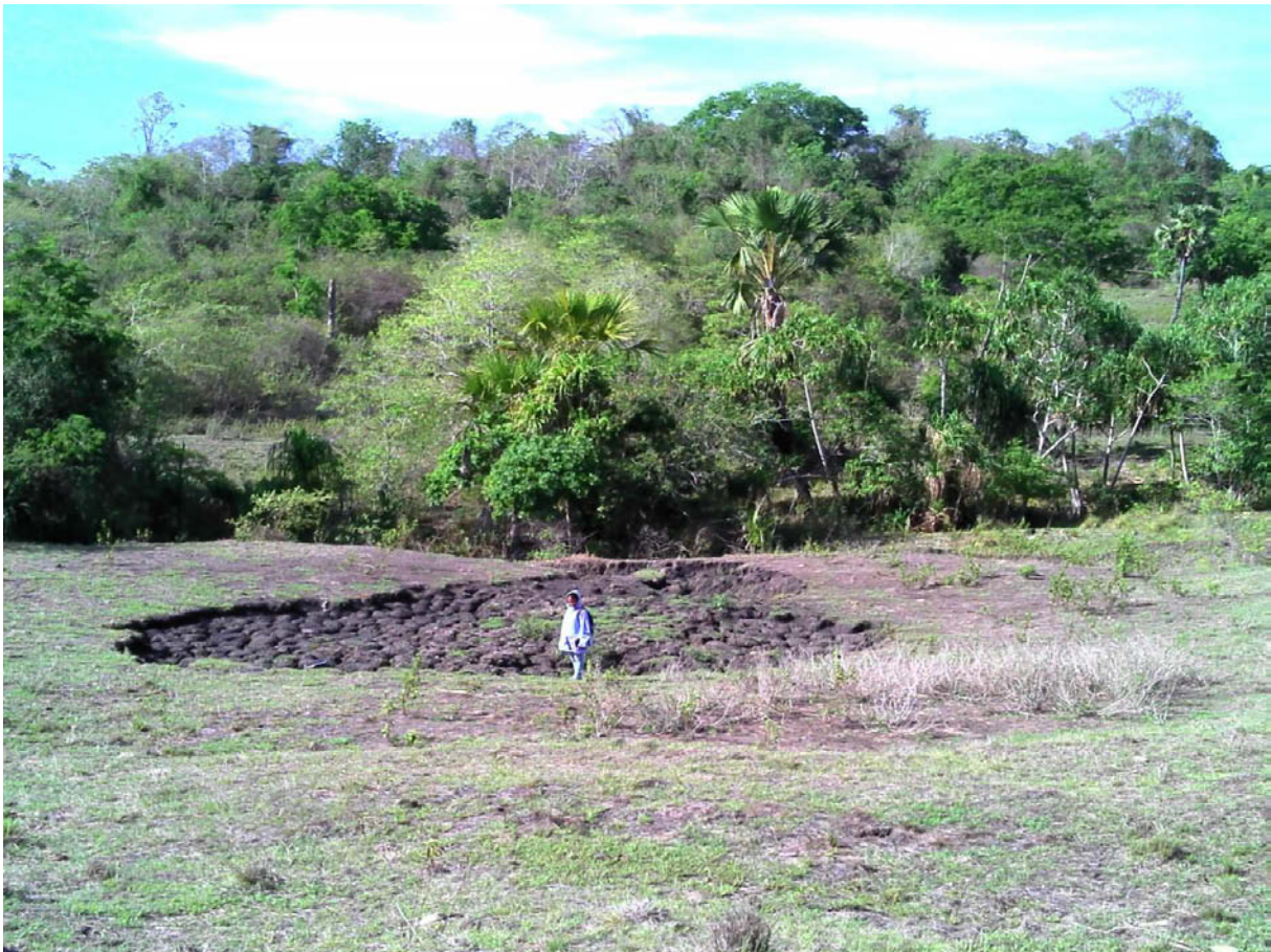
Plate 7-38 Erosion of the clayey cover material overlying the Baucau Limestone at Nova Beaco
