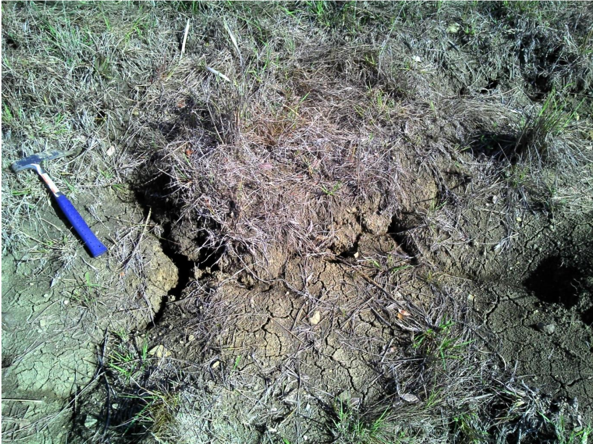
Plate 7-37 Shrinkage fissures and dispersive piping in the Bobonaro Scaly Clay Formation
