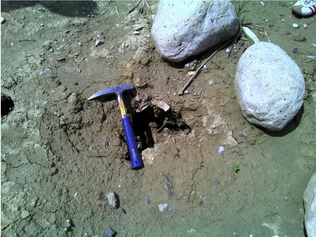
Plate 6-36 Piping features noted along the paved road bisecting Nova Betano
