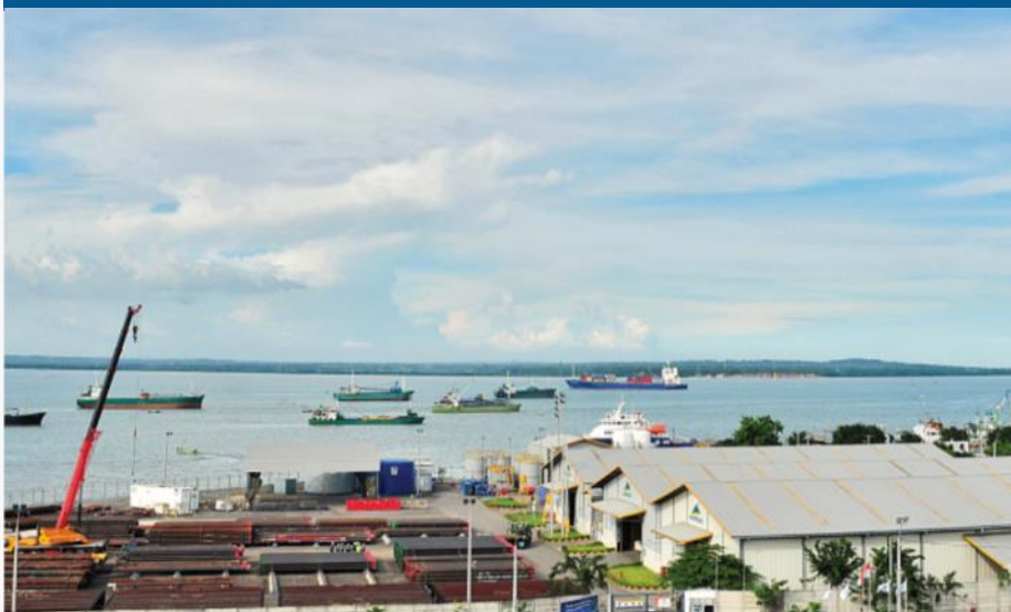
Pipe racking, fuel tanks and warehouses
