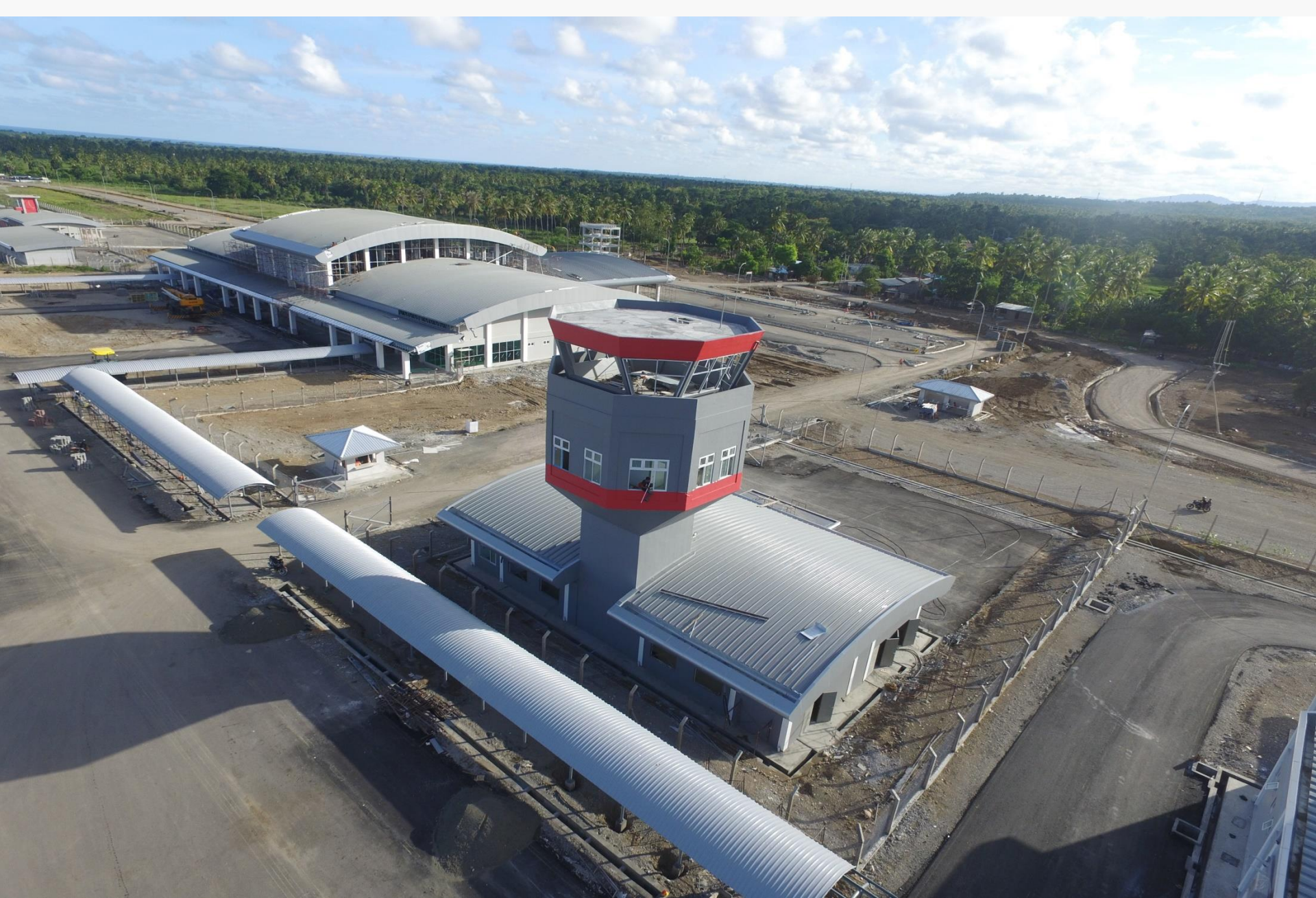
View of ATCT Building
