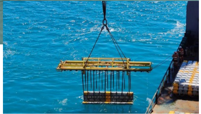
Installation of concrete mattresses for pre-lay span supports within Darwin Harbour.
