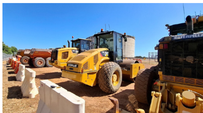
Plant equipment at DLNG preparing for shore crossing construction.
