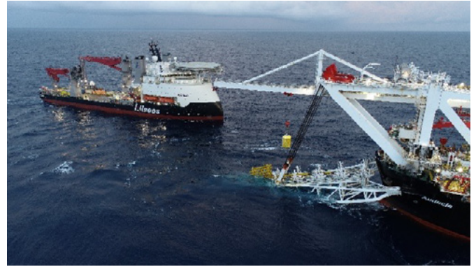
Installation of the GEP by the 'Audacia' (below), supported by the 'Fortitude' (above) construction support vessel.
