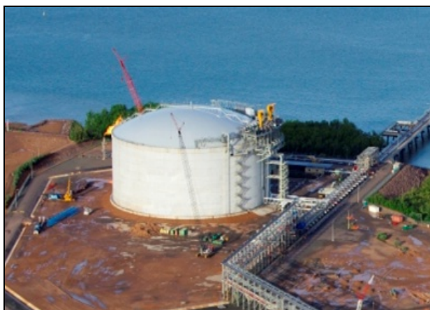
Figure 9. Standing nearly 47 m high, the LNG storage tank in Darwin can store 188,000 m 3 of gas. [13]
