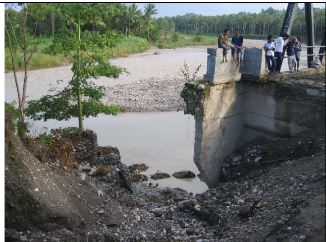
Figure 33. Collapse of the road embankment. The structural remains show a lack of transition slab, an insufficient flange length, inappropriate drainage, and poor embankment erosion protection at its base by the river. A temporary repair was made five months after the bridge collapsed, slightly widening the roadway so that four-wheeled vehicles could cross. It took another year, until October 2007, before the national government permanently repaired the bridge.
