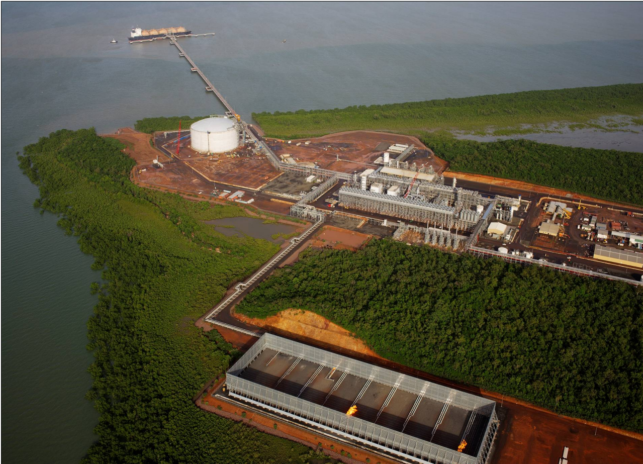
Figure 6. The Darwin LNG plant which processes gas from Bayu-Undan. [18] The jetty to the LNG tanker is 1.3 km long.
