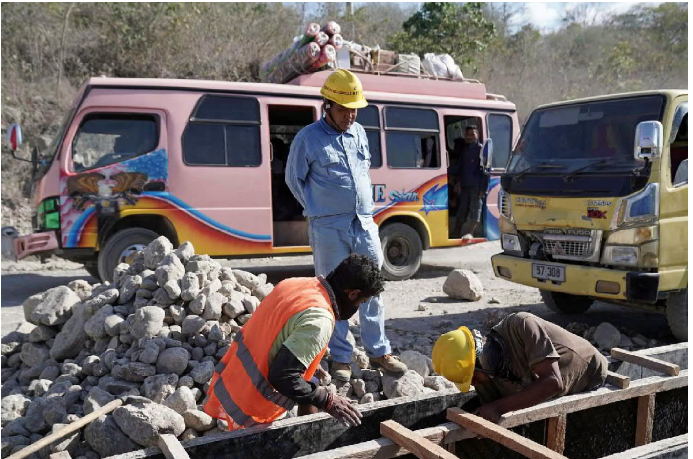
A Chinese worker supervises construction in Laleila.
