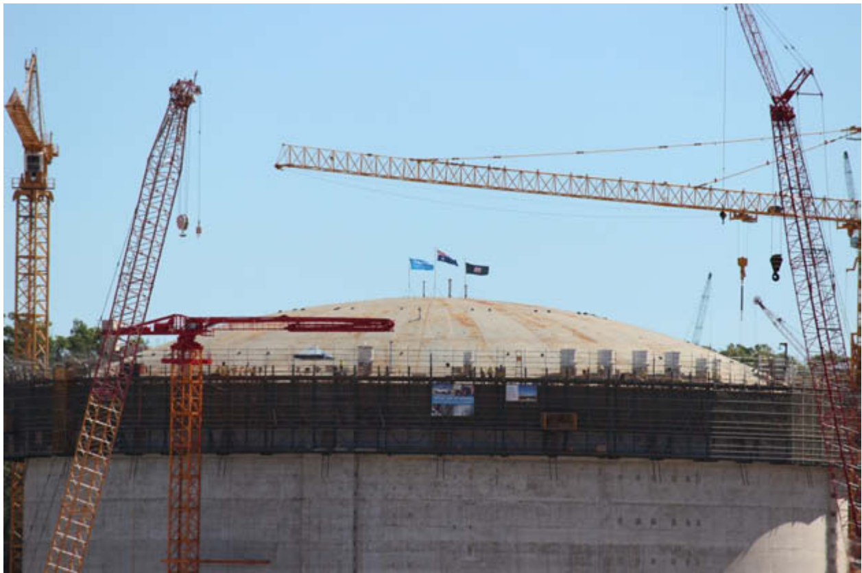
Roof raised at LNG Tank B on Curtis Island, June 2013.
