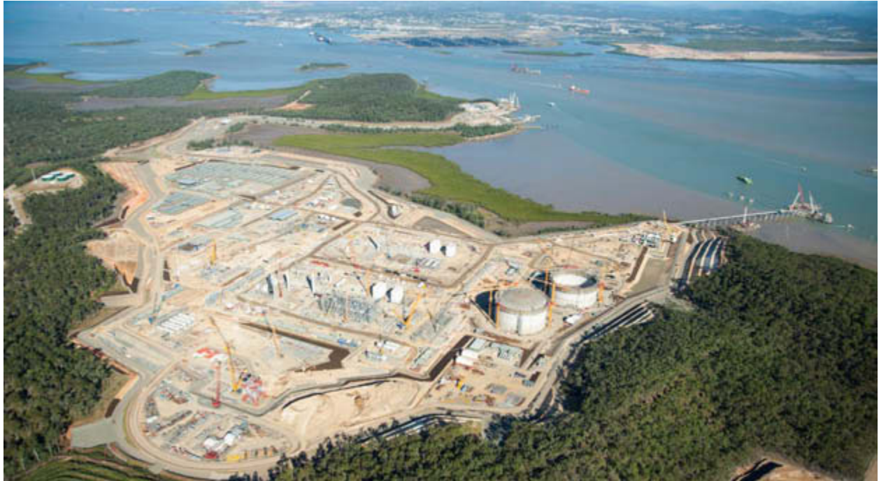
LNG plant site on Curtis Island, June 2013.
