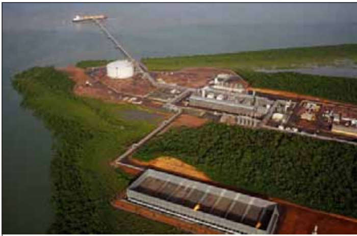
Fabrika Wickham Point LNG ne'ebe liquifika ga natural hosi Bayu-Undan. Ponte-kais nia distansia maizumenus kilometru 1.3, tanke armajen nia aas metro 45, no fabrika harii iha fatin luan hanesan ho kampu futebol 30 nia laran.
